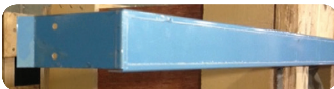
Figure 14. Roof Rib Cap
