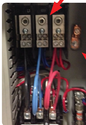
Figure 23-1. Power Distribution Block
