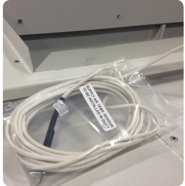
Figure 16. Duct Connection – SA Temperature Sensor
