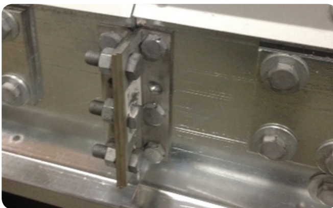
Figure 13. Outside Join Section Base Angle
