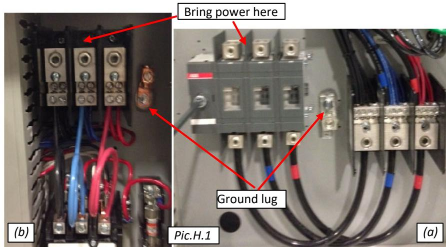
Dehumidifier with Electric Heater - Single- and Dual-Point Power Connection.
