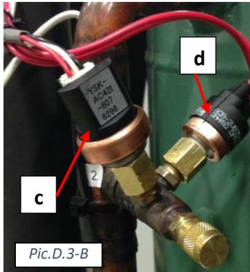
Compressor operation is monitored with **pressure sensors** (Pic. D.3-B):
